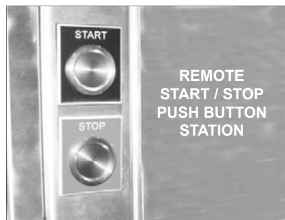
A Remote Start/Stop Station is located on the load-end of the dishwasher.
