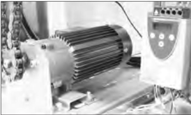
Variable Frequency Drive (VFD) Conveyor Drive Motor
