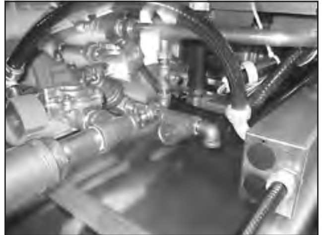
Hot water connection
