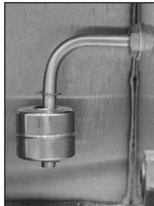
Figure 12 Float Switch
