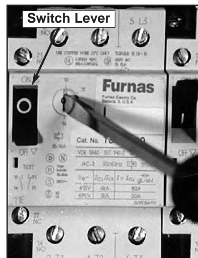
Figure 10 Motor Overload
