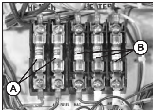
Figure 9 Fuses (Three phase shown)
