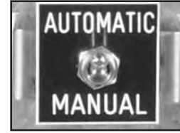
Figure 14 Bypass Switch
