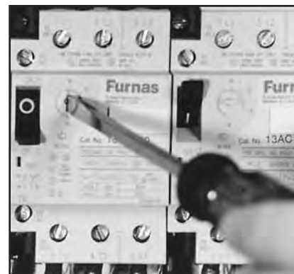
Figure 10 Motor Starter Overload
