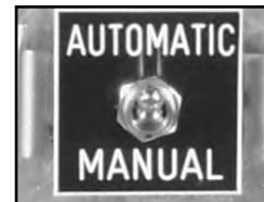
Figure 17 By Pass Switch
