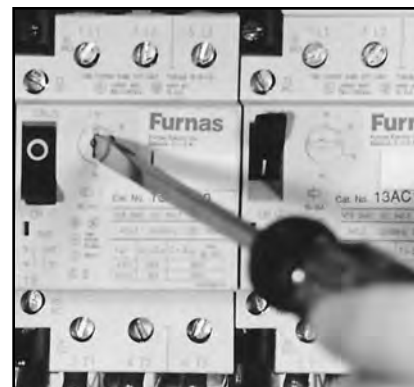
Figure 10 Motor Starter Overload
