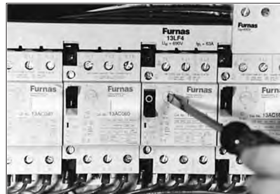
Figure 3 Motor Overloads
