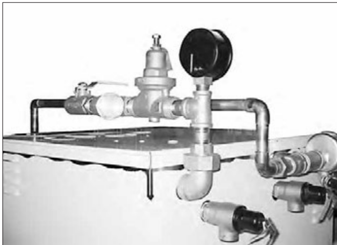
Disconnect Existing plumbing from the CH-60 booster.
