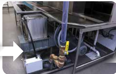
SHREDDER W/ PIPE TO CENTRIFUGE
