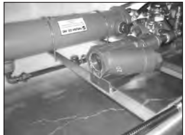
Steam and condensate connection
