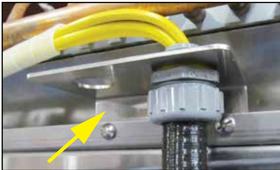
Fig. 3 - Compressor Cable Bracket
