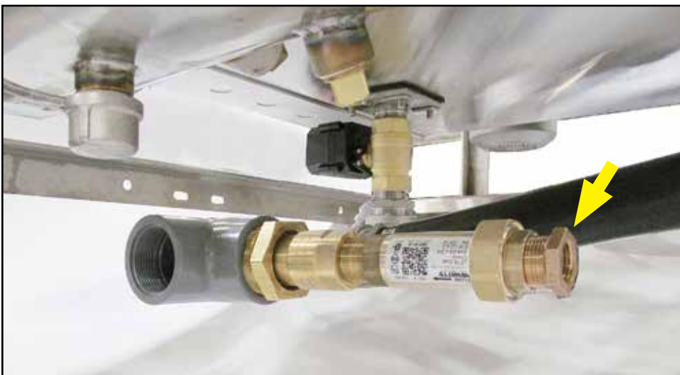
Fig. 6 - Mechanical DWT valve.
