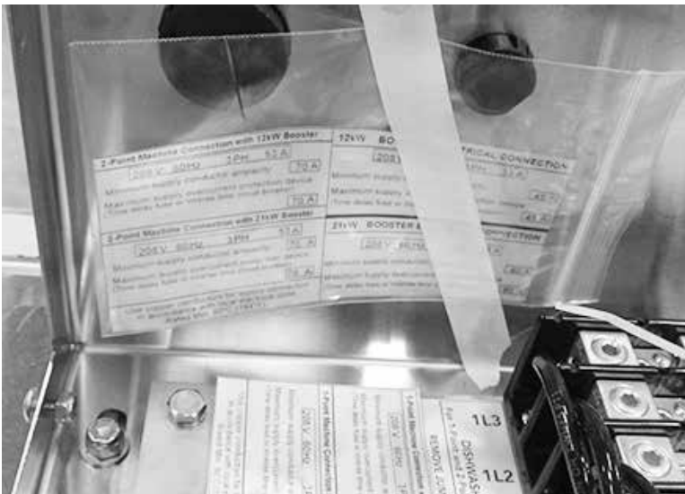
Fig. 25 - The 2-point data plate is located in a plastic bag next to the terminal block.
