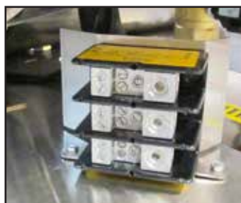
Fig. 3 - Booster terminal block
