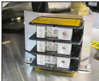
Fig. 3 - Booster terminal block
