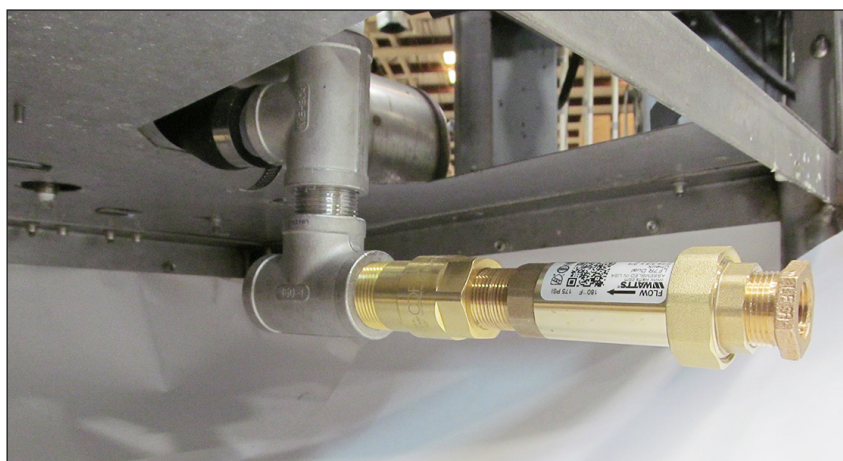
Fig. 8 - Mechanical drain water tempering valve
