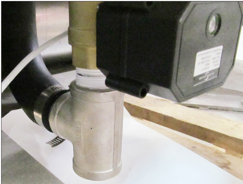
Fig. 7 - 1" NPT electric drain valve connection
