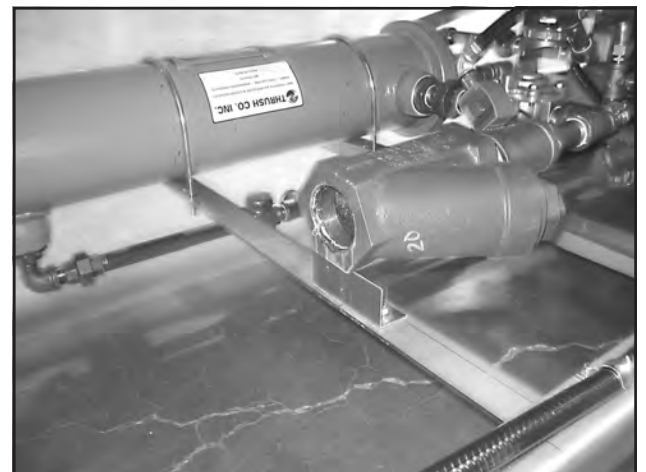
Steam and condensate connection
