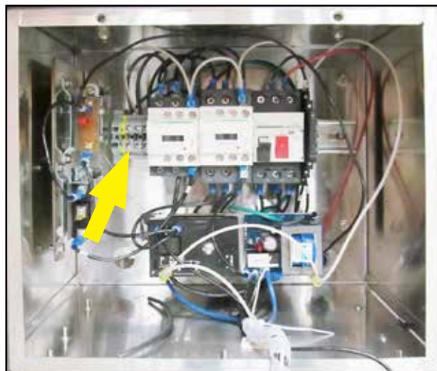
Fig. 9 - Input terminal block.
