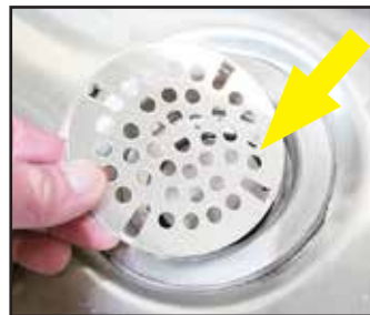
Fig. 15 - Check drains seats and screens. Ensure putty has been removed from drain clamping ring.
