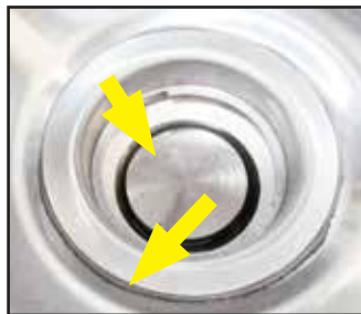
Fig. 15 - Check drains seats and screens. Ensure putty has been removed from drain clamping ring.
