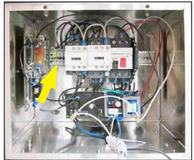
Fig. 9 - Input terminal block.
