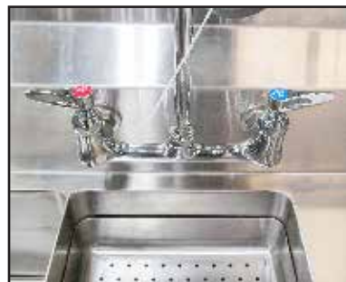
Fig. 4 - Sample pre-rinse sprayer install.
