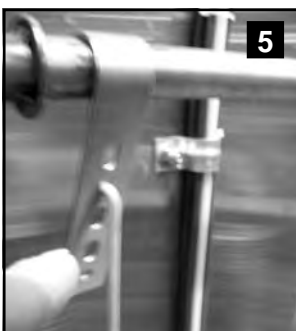
Adjust Door Spring Tension
