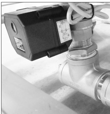
Fig. 6B - Electric Drain Valve
