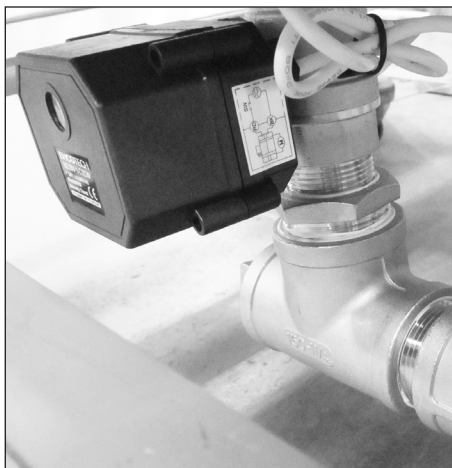
Fig. 6B - Electric Drain Valve
