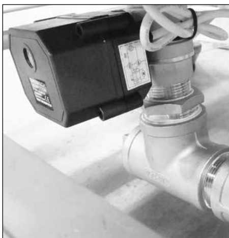
Fig. 6B - Electric Drain Valve
