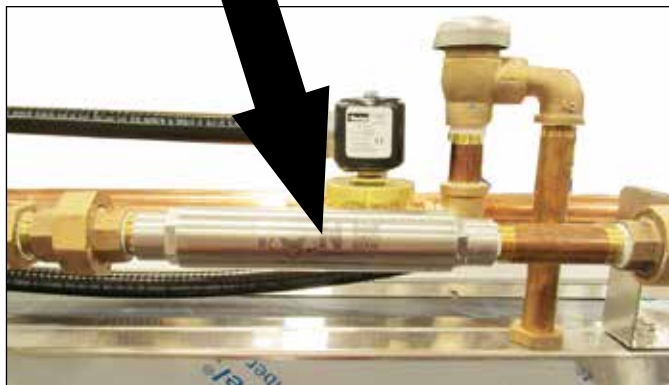
Fig. 7b - Ion Water Conditioner Installed
