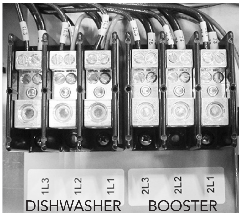
Fig. 27 - Input power is a split connection.
