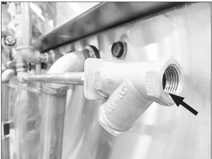
Fig. 17 - Hot water connection.
