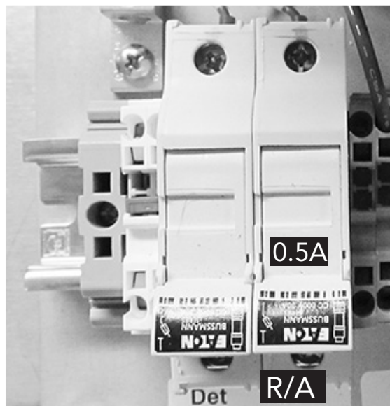
Fig. 25 - Rinse-Aid signal (0.5 A fuse).
