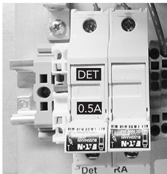
Fig. 23 - Detergent signal (0.5 A fuse).
