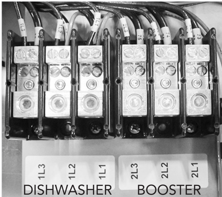
Fig. 27 - Input power is a split connection.
