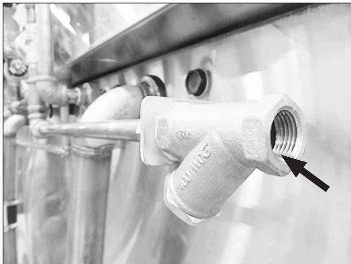
Fig. 17 - Hot water connection.
