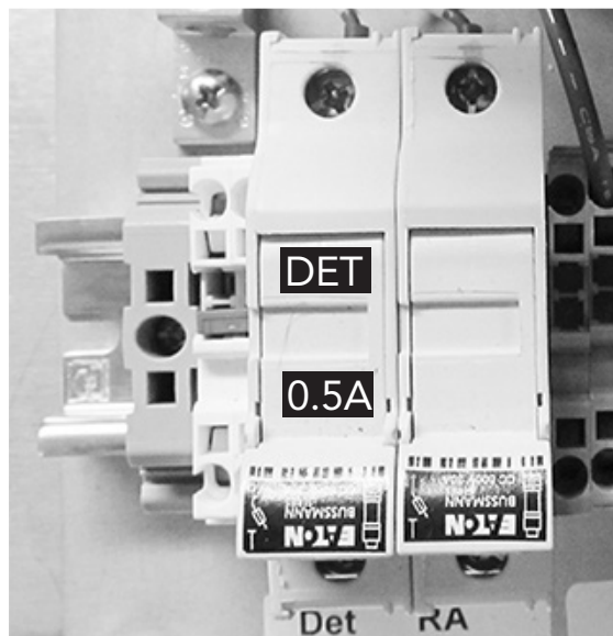
Fig. 23 - Detergent signal (0.5 A fuse).
