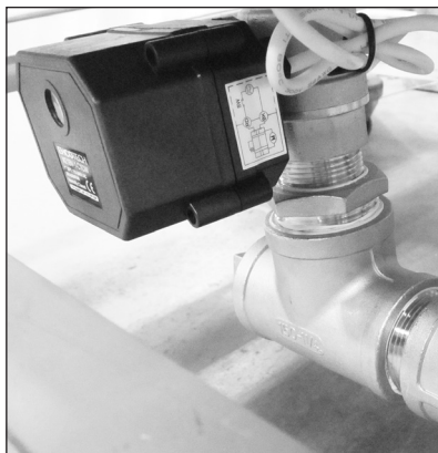
Fig. 6A - Electric Drain Valve
