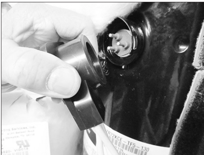
Fig. 7 - Connection is behind the insulation.
