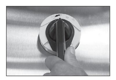
3. Engage the handle lock and insert a locking device to prevent the Breaker Switch from turning. Attach a tag on the Breaker Switch to indicate that work is being performed on the circuit.
