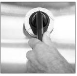
Main Circuit Breaker Switch in the OFF position
