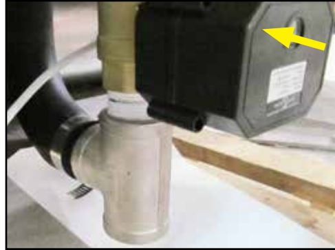
Fig. 1 - Dishwasher Drain Valve
