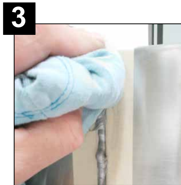
Fig. 6 - Apply sealant to the hood seams.
