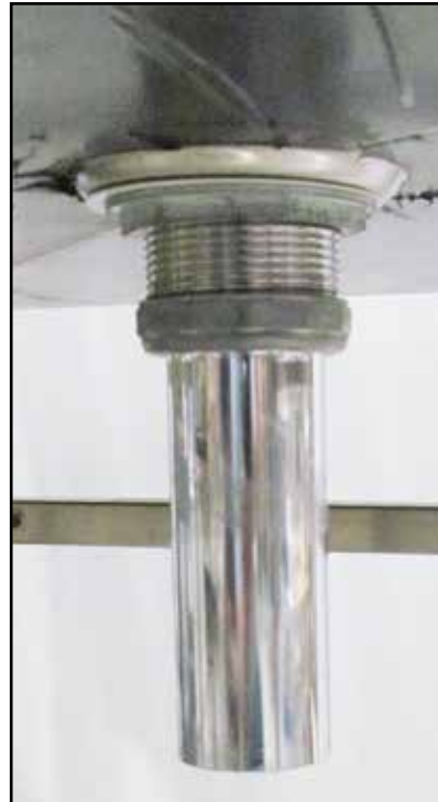
Fig. 15 - 1-1/4" slip-fit connection
