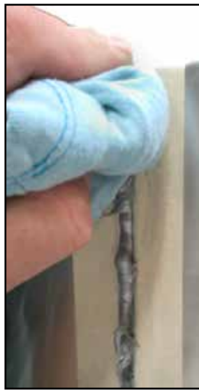
Fig. 13 - Smoothly remove excess sealant.
